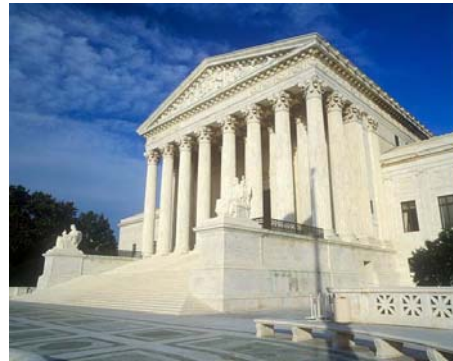
Cass Gilbert, US Supreme Court Building, Washington DC (1928 - 1935)
